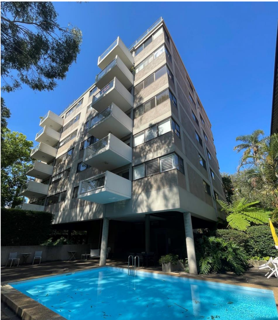
Figure 12. Rear view of 1–5 Clement Street showing pool, deep projecting balcony units and wrap around window elements to corners. Source. GML, 2024.
